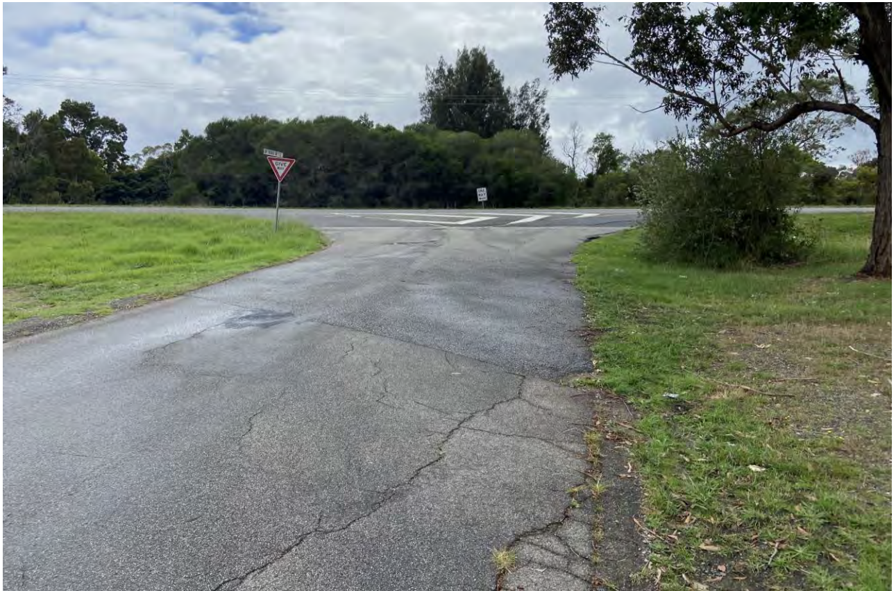
Figure 6: Sir Thomas Drive – looking north towards Princes Highway
