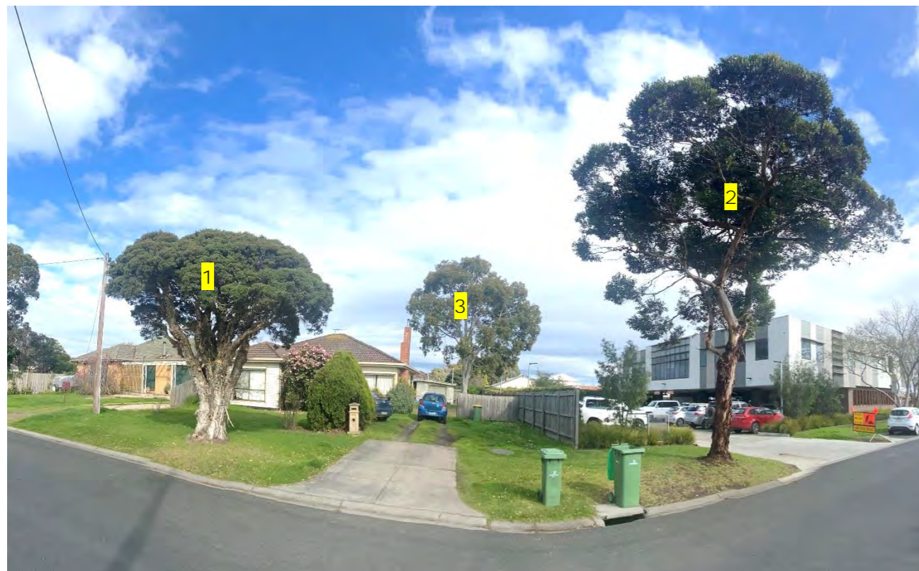
Image 2: 2 John Street frontage.
