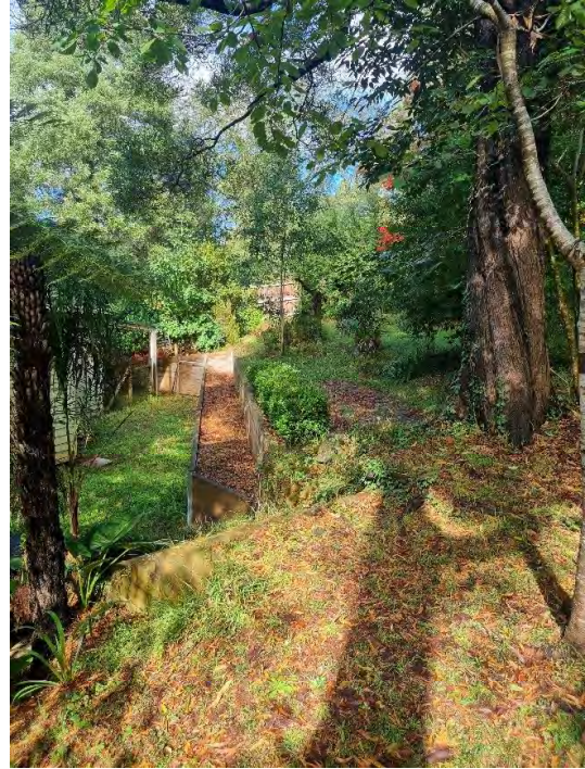
Photograph 2: Existing retaining wall to north of dwelling
