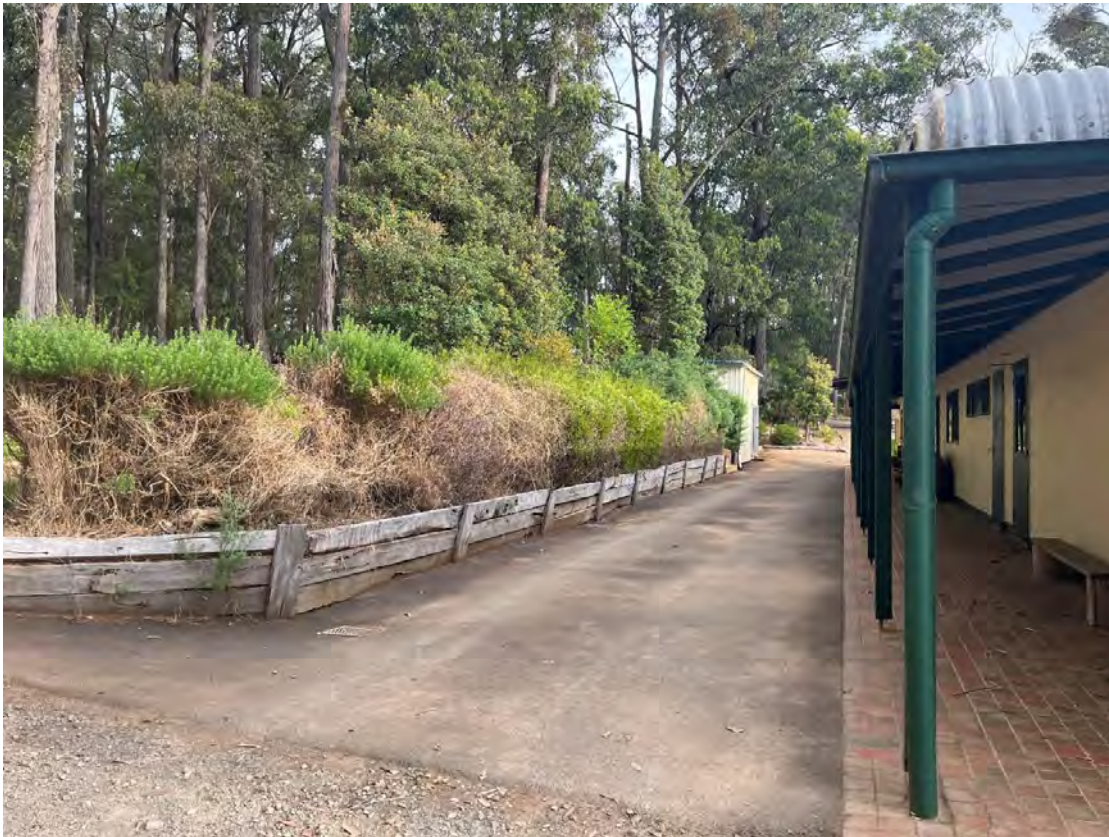
Figure 4.5. Front (NE) side of existing building. All ground cover to be removed.
