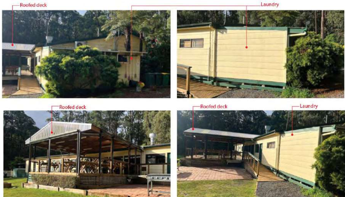
Figure 7: Images depicting roofed-deck and laundry
