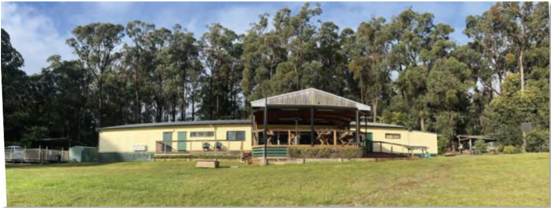
Figure 2: View to existing building, looking north
