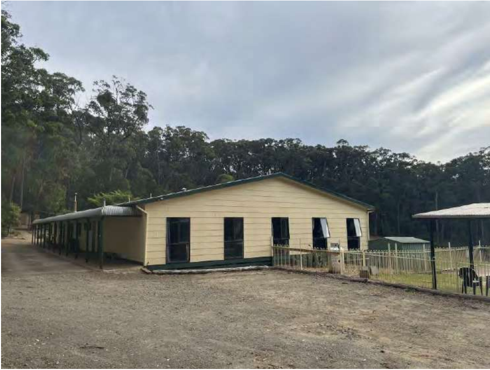
Figure 4.9. The existing building north corner.
