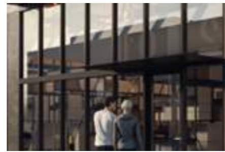
7A POWDERCOATED ALUMINIUM FRAMED WINDOW WITH CLEAR DOUBLE GLAZING FRAME : SATIN BLACK
