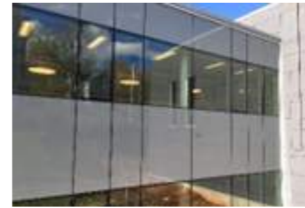
7B POWDERCOATED ALUMINIUM FRAMED WINDOW WITH COLOUR BACKED DOUBLE GLAZING FRAME : SATIN BLACK GLASS : GRAPHITE
