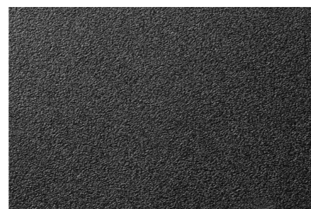
13B BITUMEN ROAD
