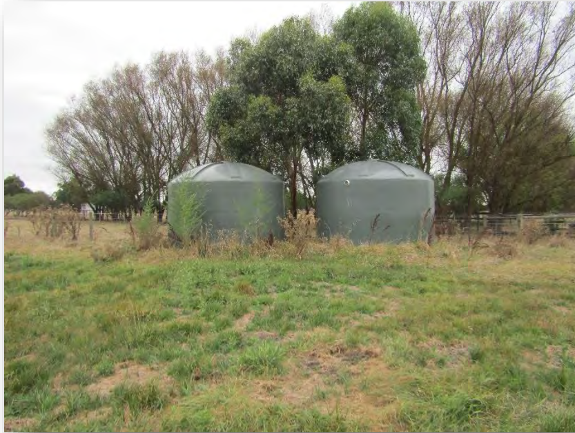
Plate 5 - Photo depicting the two 22,500L water tanks – total capacity 45,000L available for stock filled by water carrier or connected to the water bore.
