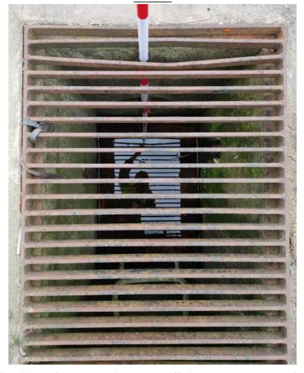
Figure 11. Depth of storm water drain (scale increments = 20cm) running along the northern side of the warehouse. Several storm water grates of similar design and depth are present across the activity area.
