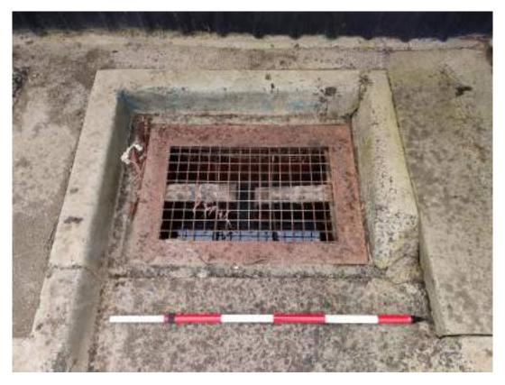
Figure 13: Truck cleaning area for collecting dirt and oil, constructed in the northern part of the site.
