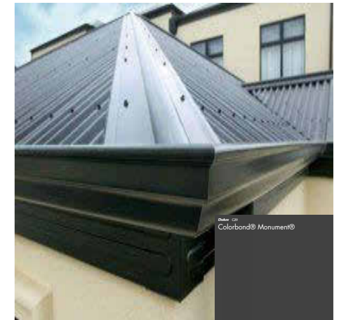
RFA-01 FASCIA: PRESSED METAL - DULUX COLORBOND 'MONUMENT' OR SIMILAR
