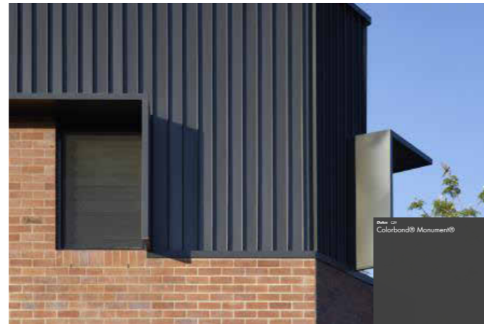
CLF-01 VERTICAL CLADDING: VERTICAL CLADDING: LYSAGHT - 'LONGLINE305' - DULUX COLORBOND 'MONUMENT' OR SIMILAR MATT FINISH
