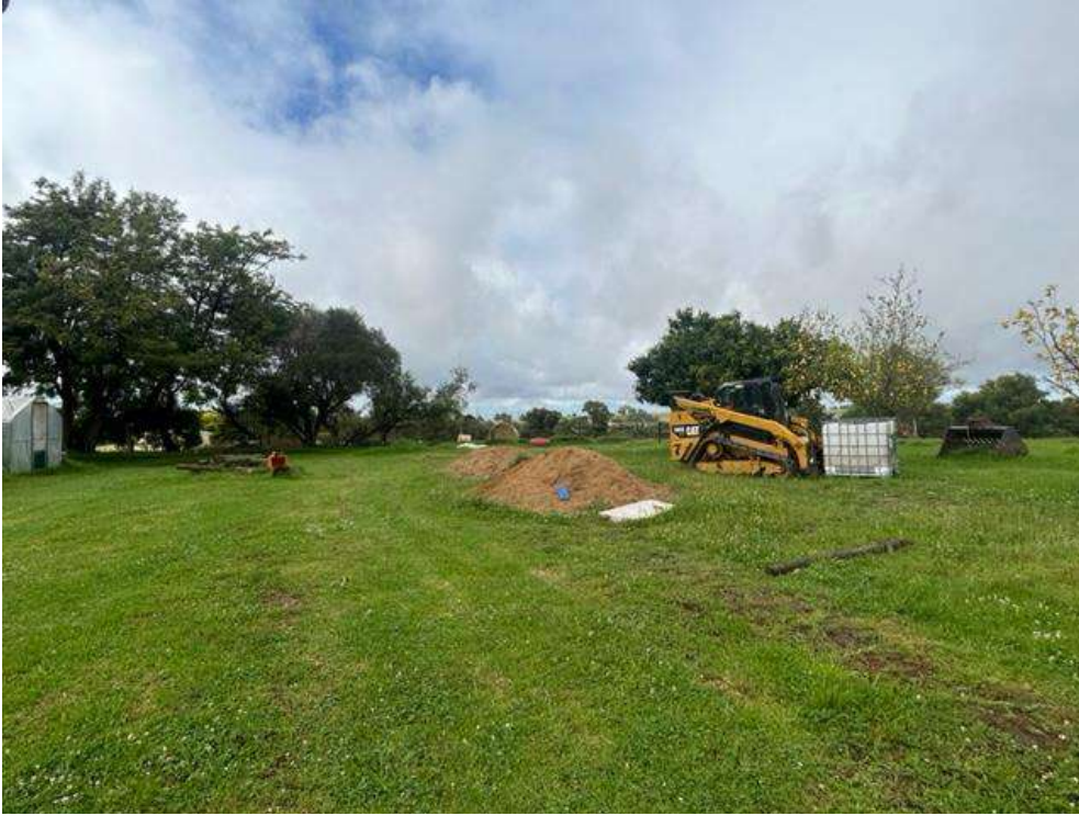
Looking south across build site
