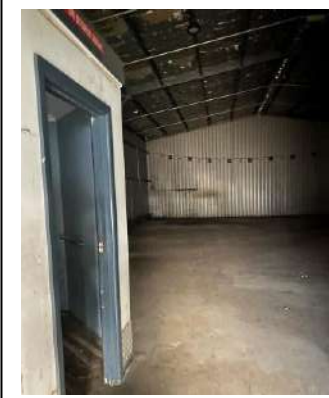
7. INSIDE WAREHOUSE 1 TO PROPOSED CAR PREP AREA AND CAR WASH BAY. THERE IS NO INTENTION TO BREAK INTO THE BOUNDARY WALL TO WAREHOUSE 2.
