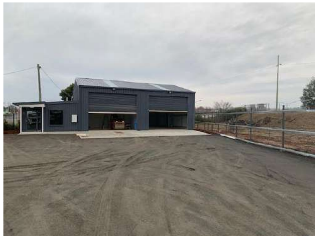
Figure 11: Interceptor outside wash bays Warragul (source Budget).
