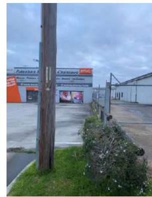
4. VIEW LOOKING SOUTH ACROSS NO. 15 & 17 BALD HILL ROAD AND SITE OF PROPOSED NEW FENCE FOR NO. 15 WILL SIT A METRE BEHIND POLE.
