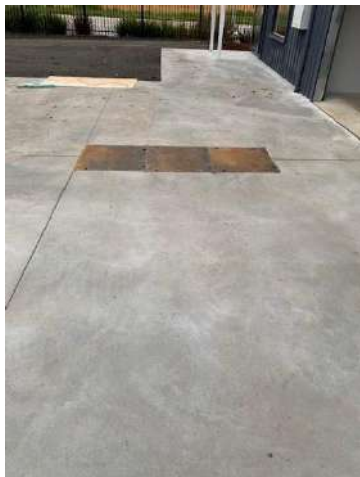
Figure 10: Interceptor at Budget Warragul (Source Budget).
