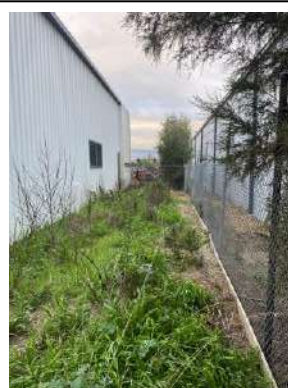
12. LOOKING EAST ALONG EASEMENT AT REAR OF 15 BALD HILL ROAD AND WAREHOUSE 3. TIE POINT LOCATED WITH PIPE ON WAREHOUSE JUST VISIBLE NEAR WINDOW TO CONNECT INTERCEPTOR.
