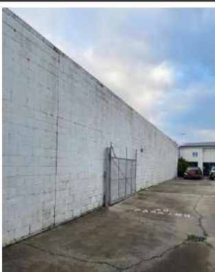
11. LOOKING EAST AT BOUNDARY WALL OF NEIGHBOUR NO. 17 BALD HILL ROAD.
