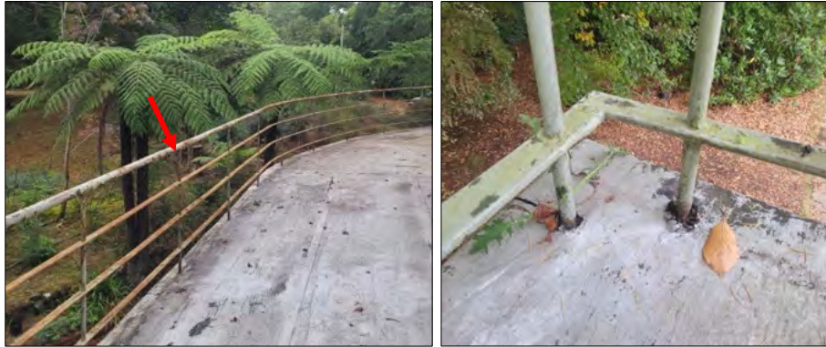
Figure 19 Detail of the condition of the existing first floor balustrade.
