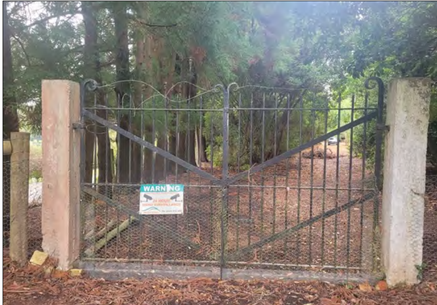
Figure 36 Existing southwest corner gates.
