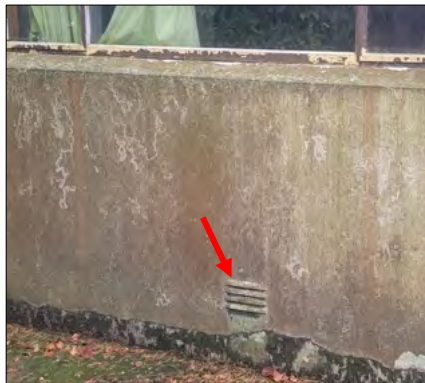
Figure 20 (left) Detail of the existing lower level vent – type A
