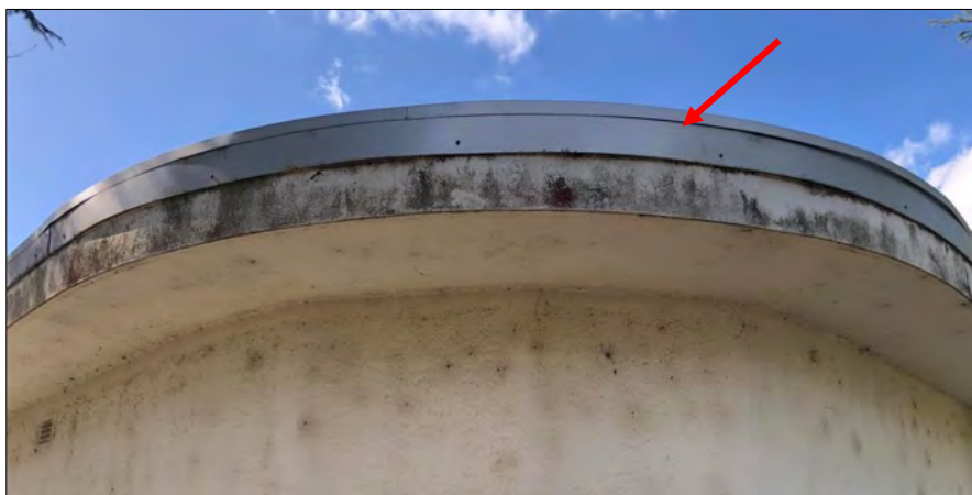
Figure 34 Detail of the modern flashing added to the first-floor roof.
