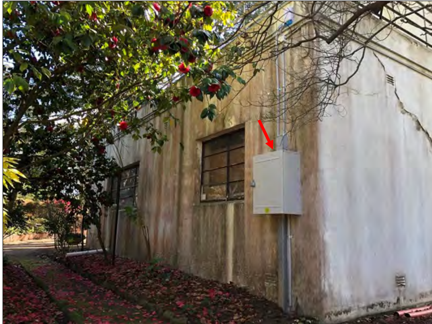
Figure 15 Existing services, conduit etc to be removed.
