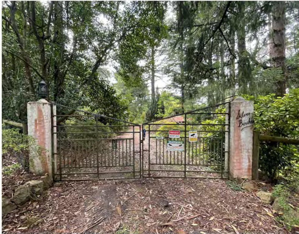
ENTRY GATE TO BE RESTORED
