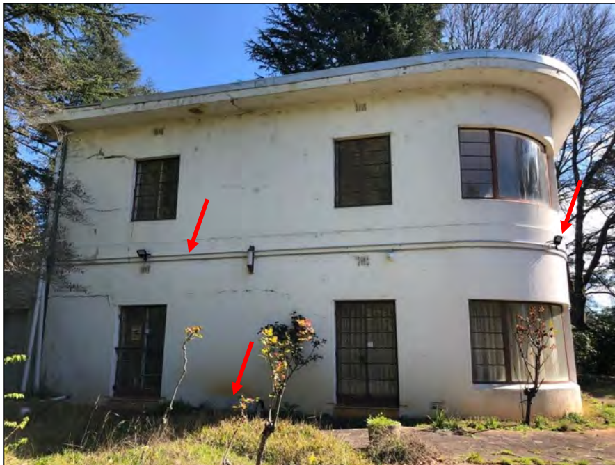
Figure 14 Existing services, conduit etc to be removed.
