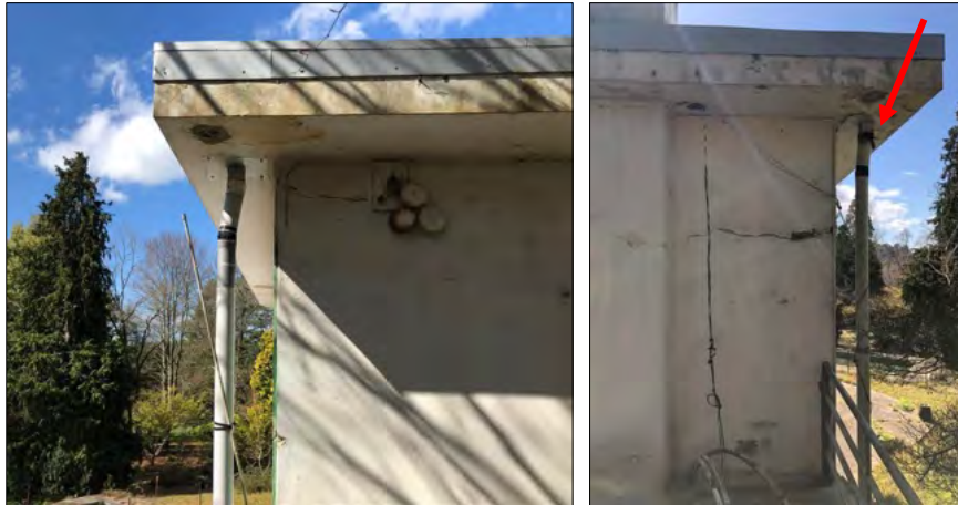
Figure 31 Detail of the various downpipes installed at the first-floor balcony.
