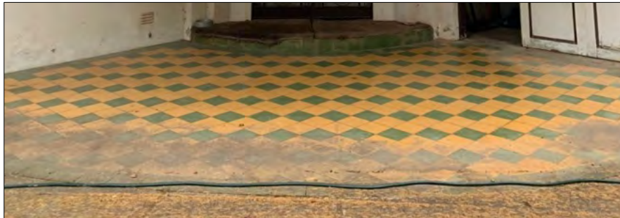
Figure 23 Detail of the existing tiling to the entrance porch to be retained and repointed.
