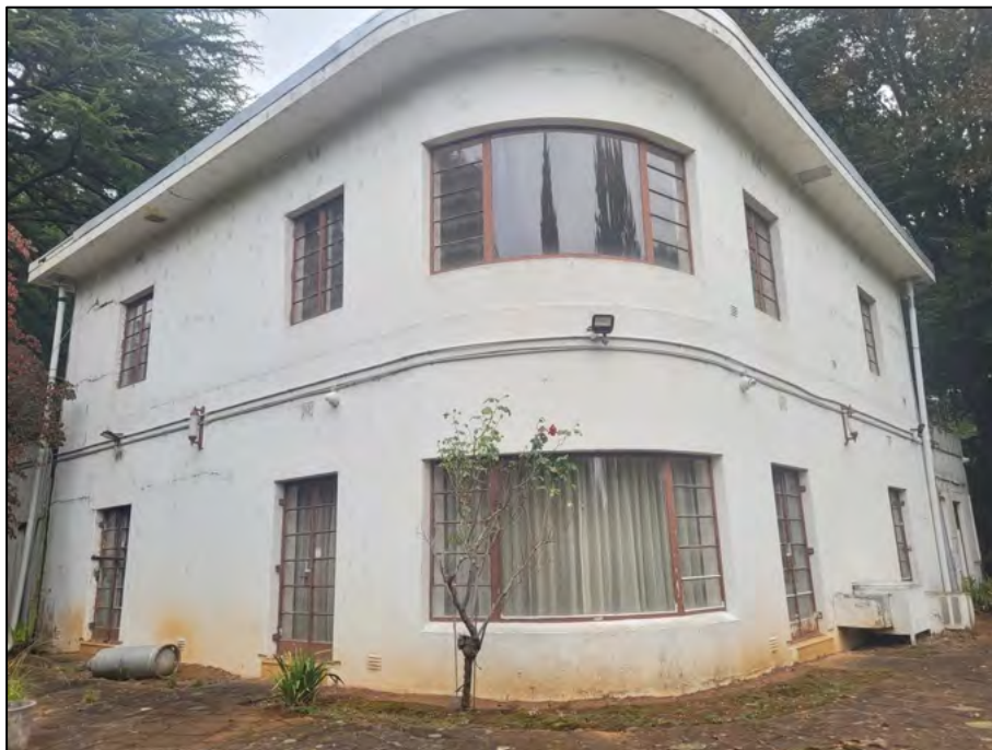
Figure 4 The rear of the dwelling as viewed from the north-east.
