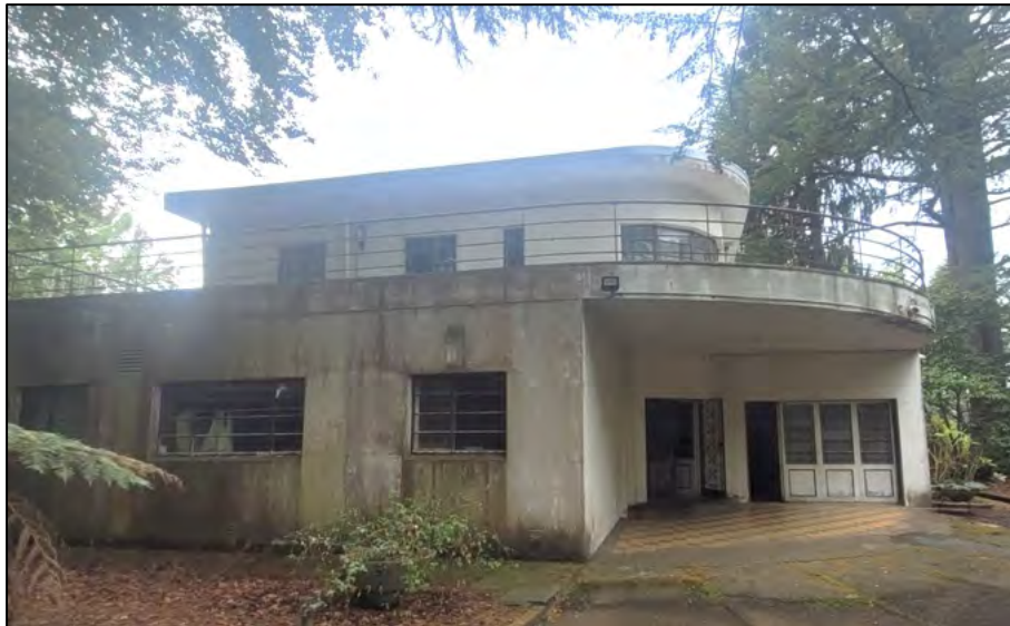
Figure 3 The c.1937 dwelling as viewed from the west.
