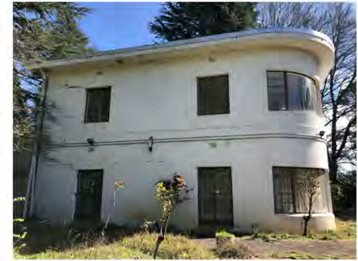
EXISTING CONDITION OF DWELLING
