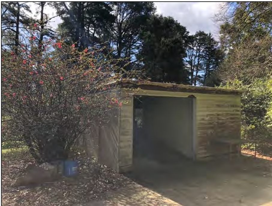
Figure 8 Shed/Garage to the west of the dwelling.
