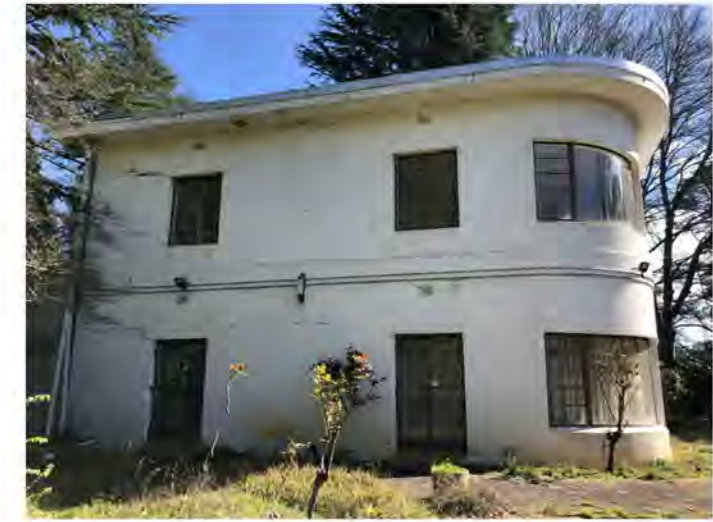
EXISTING CONDITION OF DWELLING
