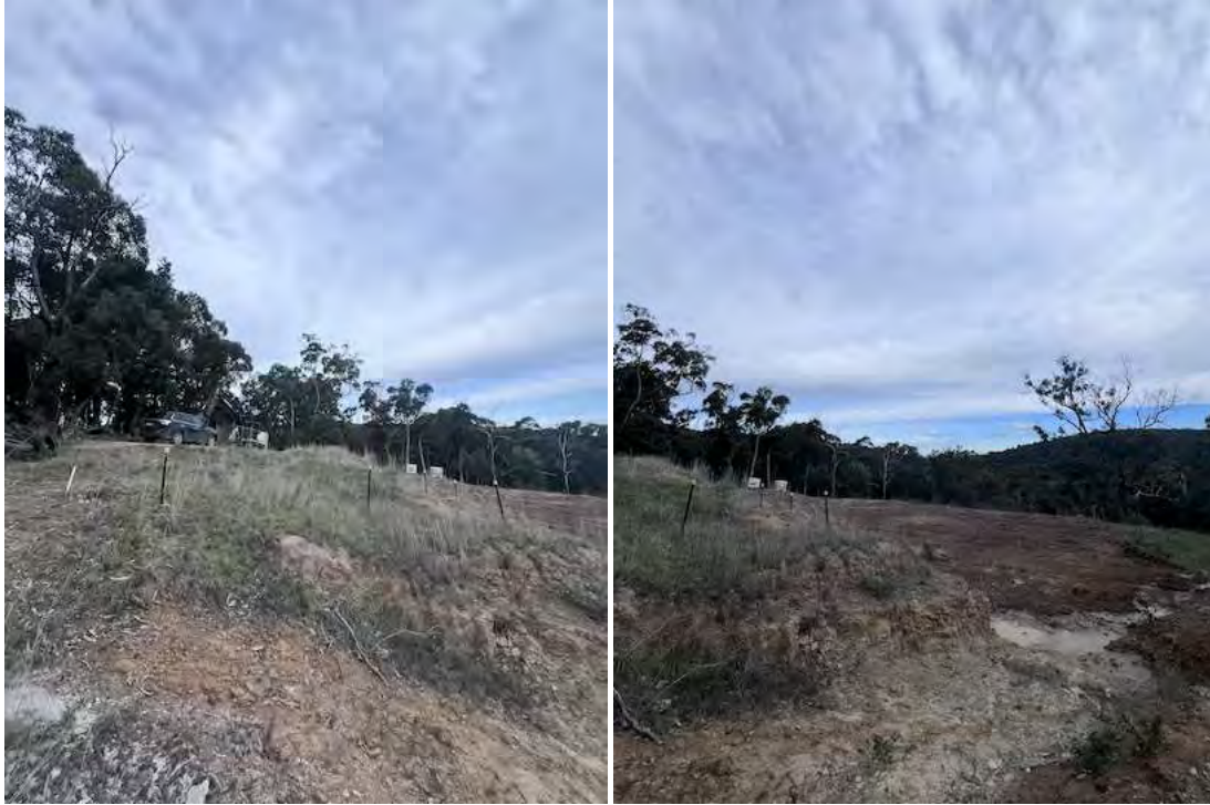
Site with existing cuts looking south with Bathe Rd entrance to the top ( Left – east)
