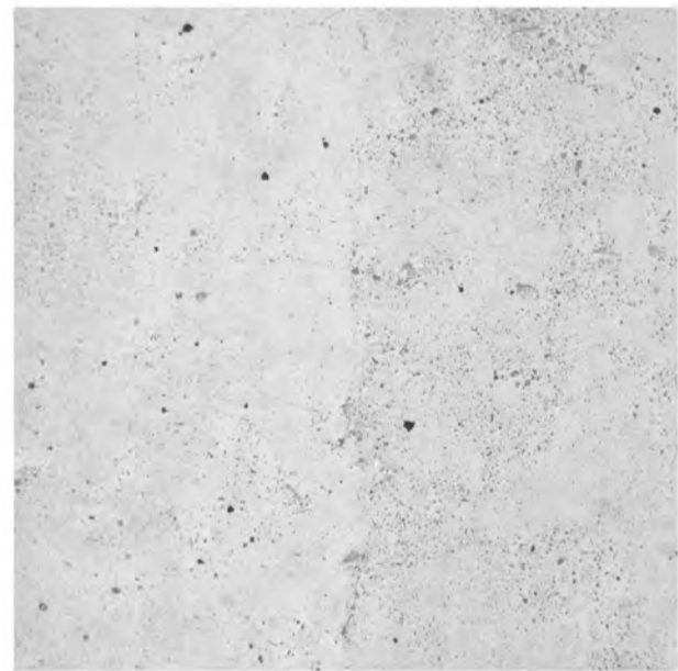
C1_CONCRETE FINISH WALLS
