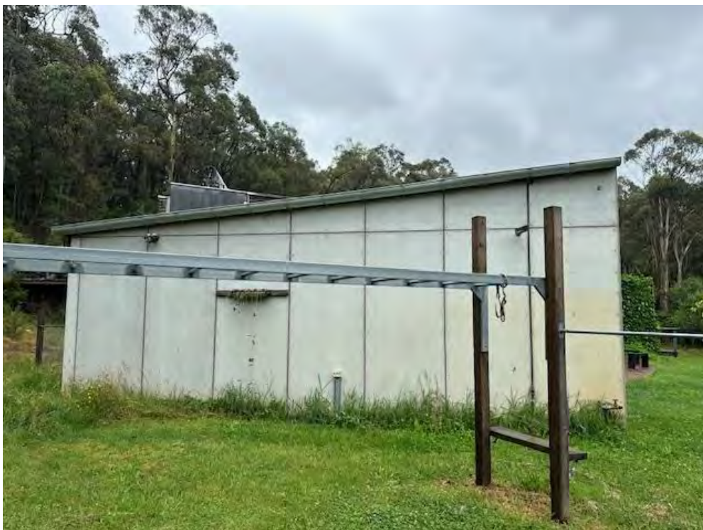
Figure 7: Rear view of the existing building (Extension starts here)
