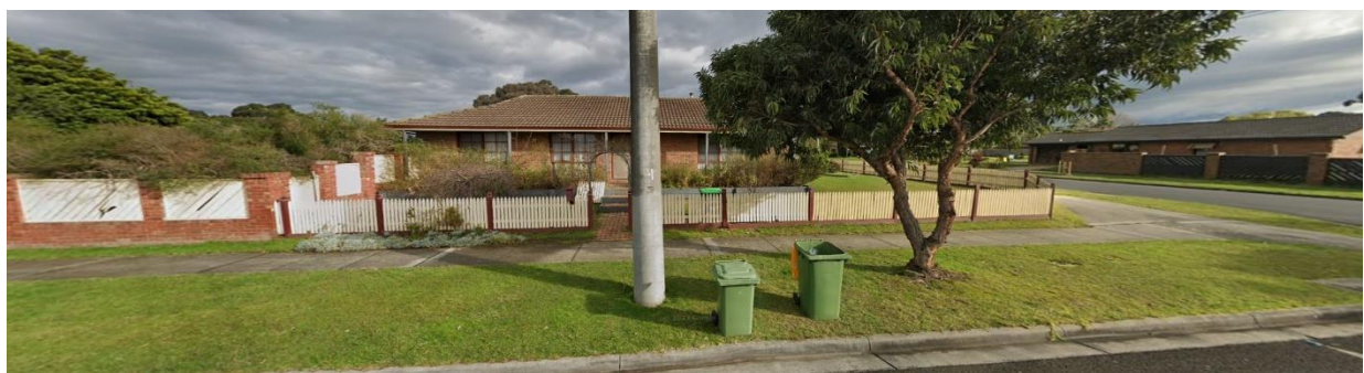
Figure 3: Street view of subject site (from Kingston Av)
