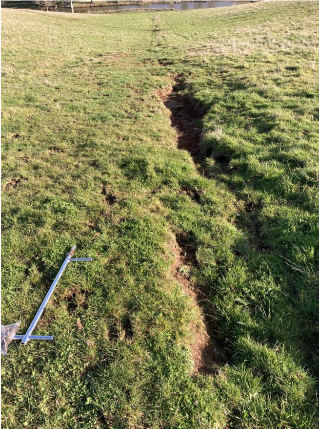
Photograph of erosion down a slope in Paddock 3 and discussed on Page 5 of this report.
