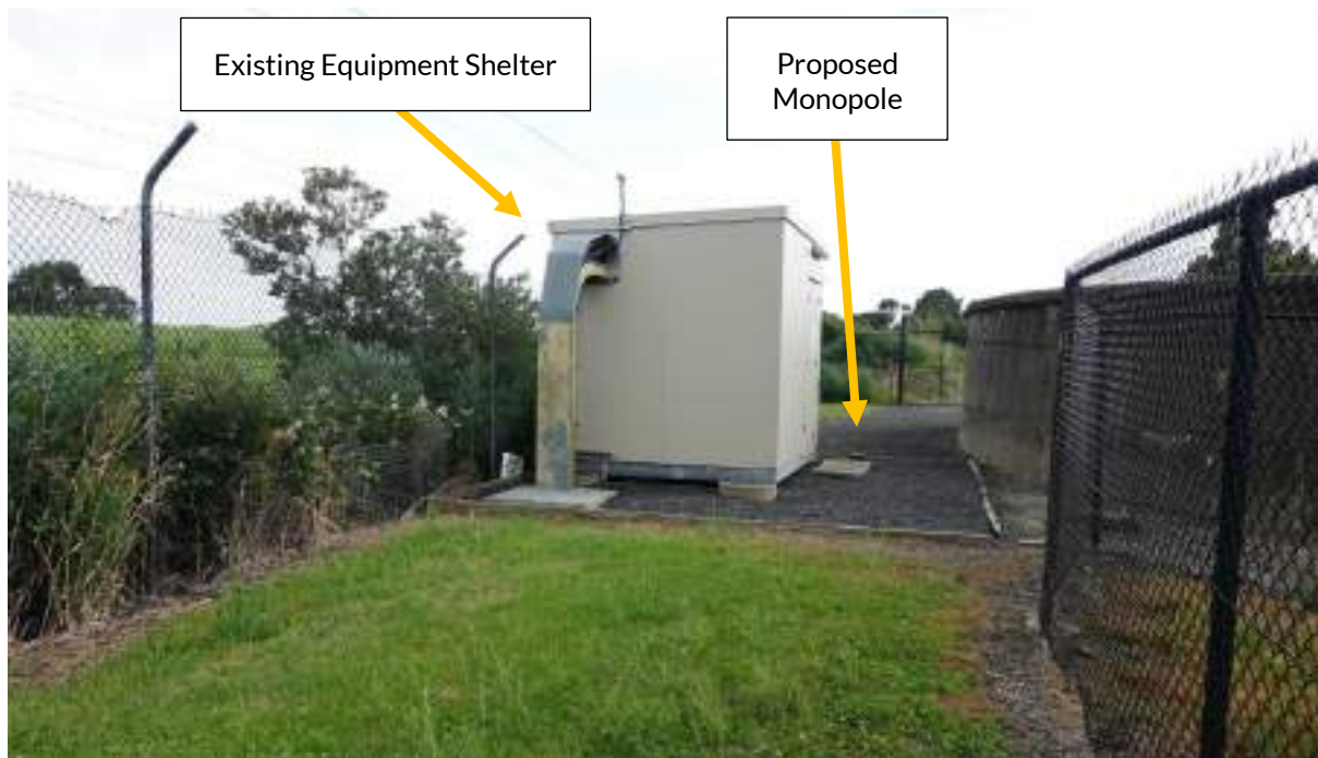
Figure 4: Northern Boundary of the South East Water Compound
