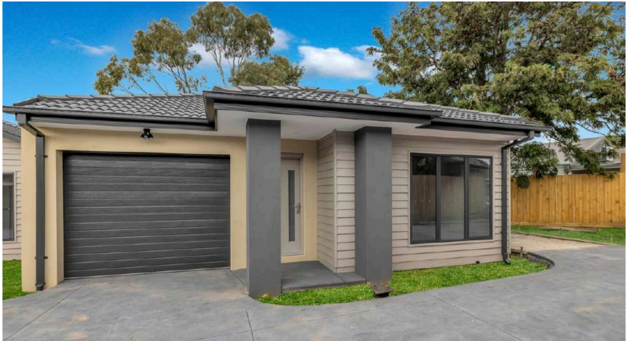
Figure 2. 6/48 James Street Facade
