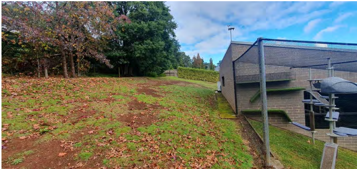
Figure 7. Existing dwelling and private open space on subject site
