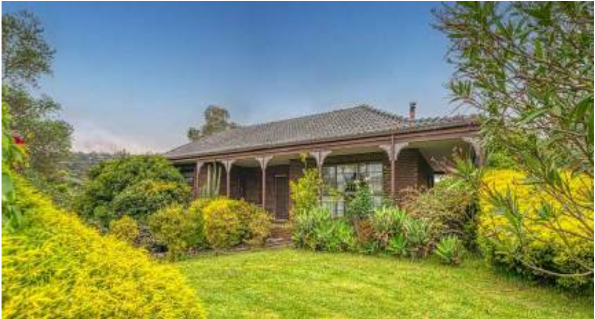
Figure 7 – Existing dwelling onsite to be decommissioned and retained.
