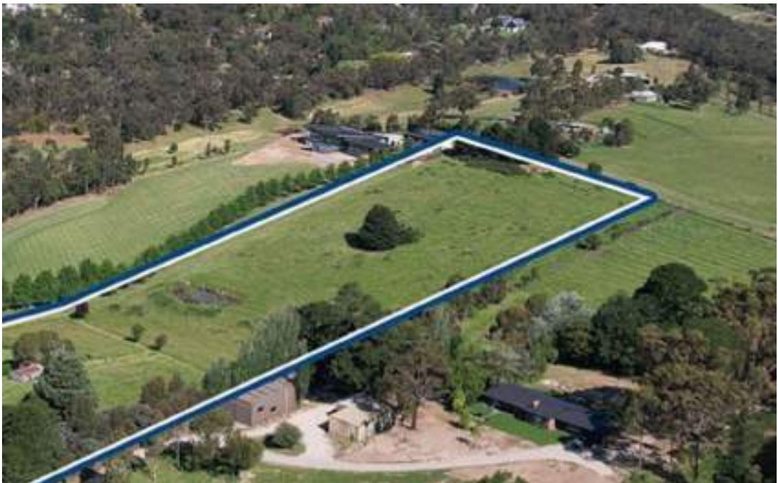
Figure 6 – aerial view of the site and adjoining developments.
