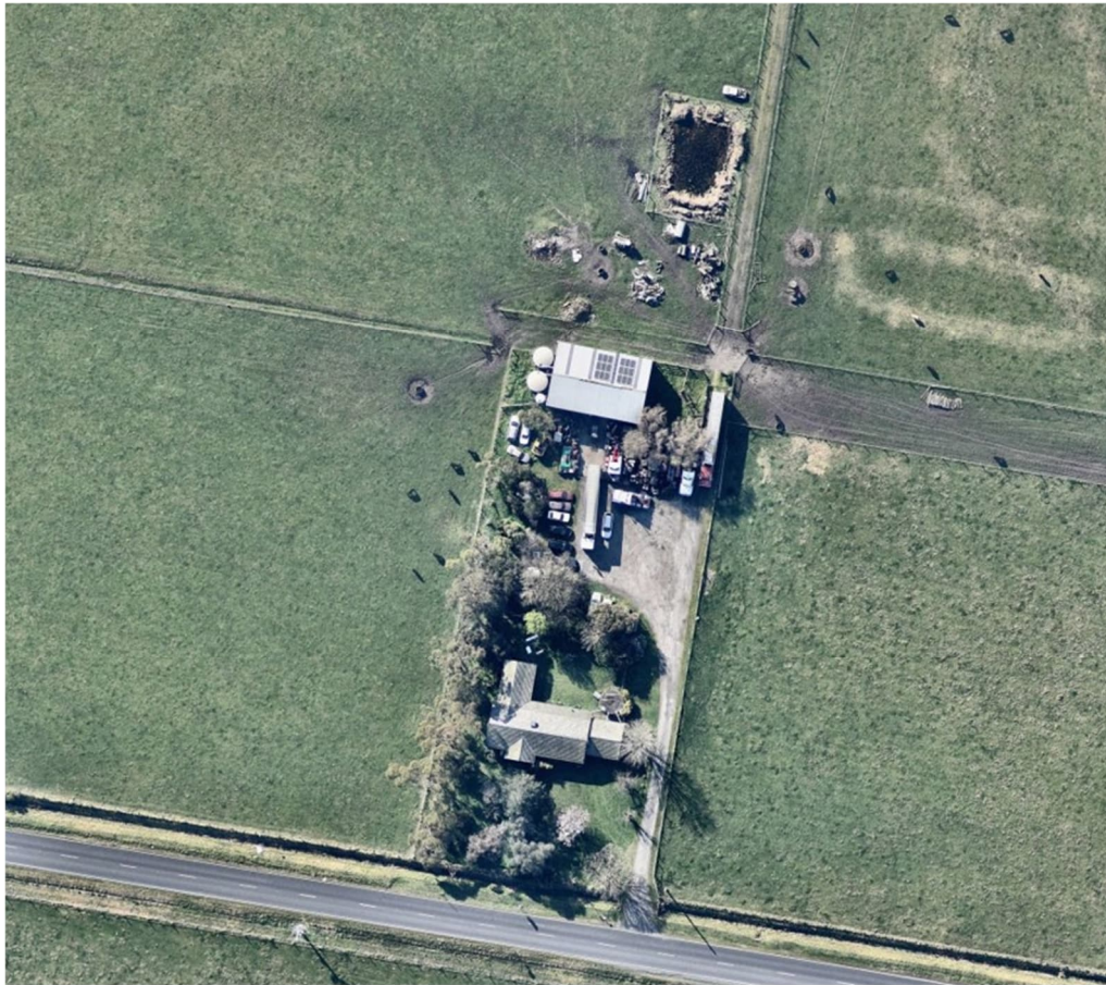
Site of proposed shed and existing buildings. Proposed shed position west of existing larger shed. (Nearmap)
