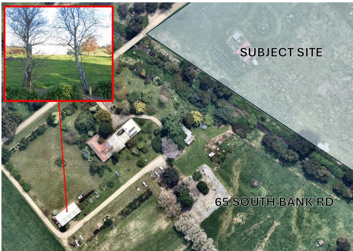
LARGE OUTBUILDING AT 65 SOUTH BANK RD
