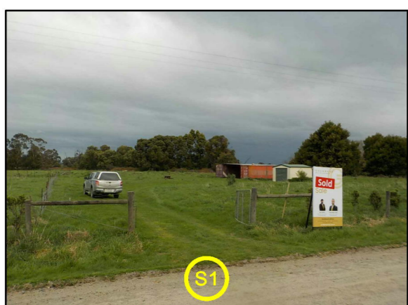
Photo # 2: South Bank Road, BUNYIP SUBJECT PROPERTY. COMPLETED SHED.
