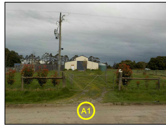
Photo # 1: South Bank Road, Bunyip ADJOINING PROPERTY. COMPLETED SHED.
