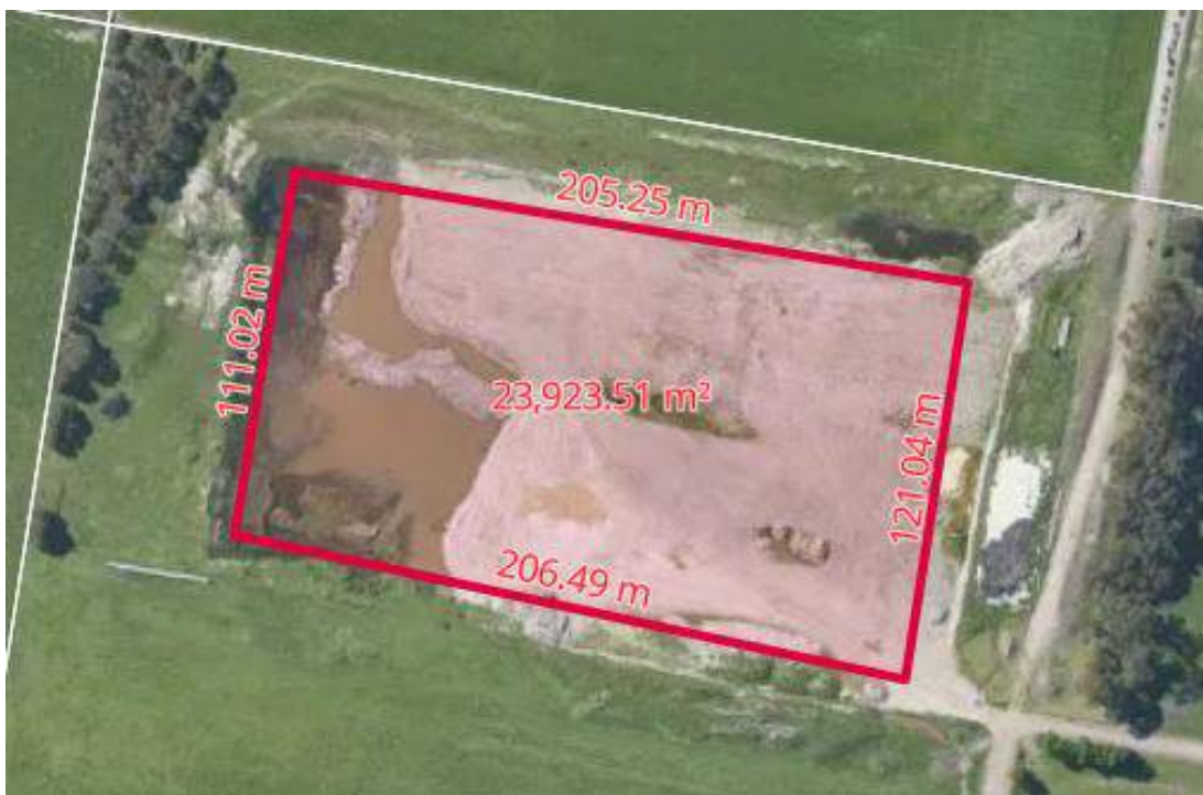
Figure 4. Dam dimensions at 105 Eight Mile Road
