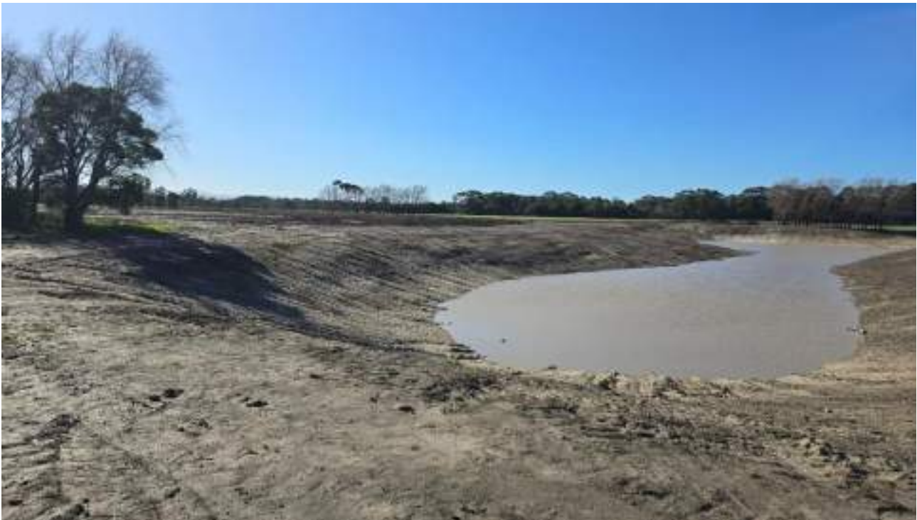
Figure 11: Site photo of dam taken at ground level
