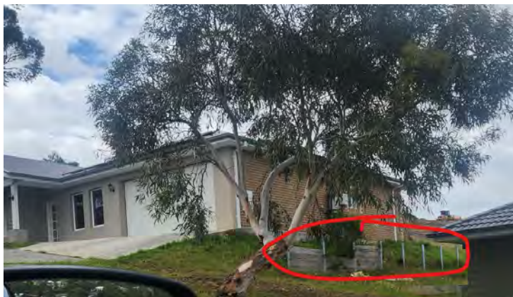
Figure 6: Examples of retaining walls use to create a flat block for ease of construction along Serene Court. Photography taken 28/11/2024 via a Samsung Phone.
