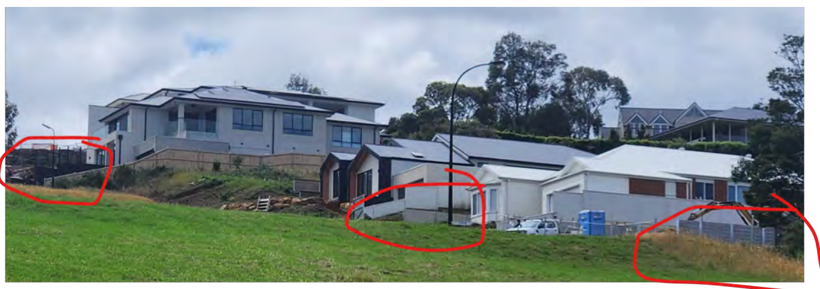
Figure 8: Examples of retaining walls use to create a flat block for ease of construction along Tranquil Way. Photography taken 28/11/2024 via a Samsung Phone.
