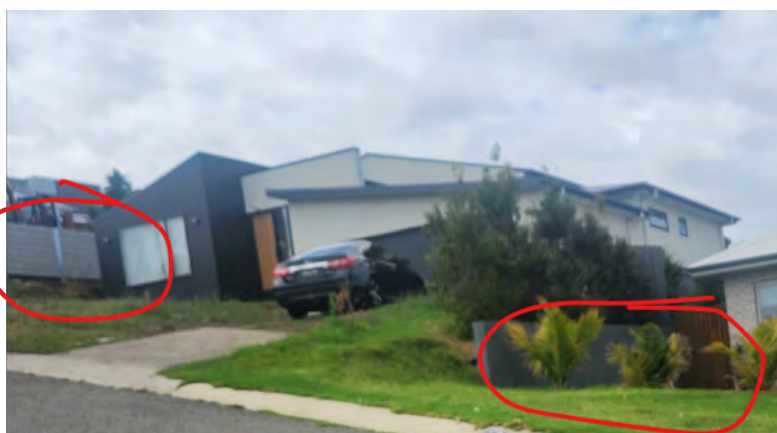
Figure 7: Examples of retaining walls use to create a flat block for ease of construction along Tranquil Way. Photography taken 28/11/2024 via a Samsung Phone.
