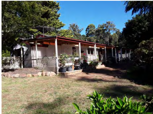
LOOKING SOUTH FROM BACK YARD TO REAR OF EXISTING DWELLING
