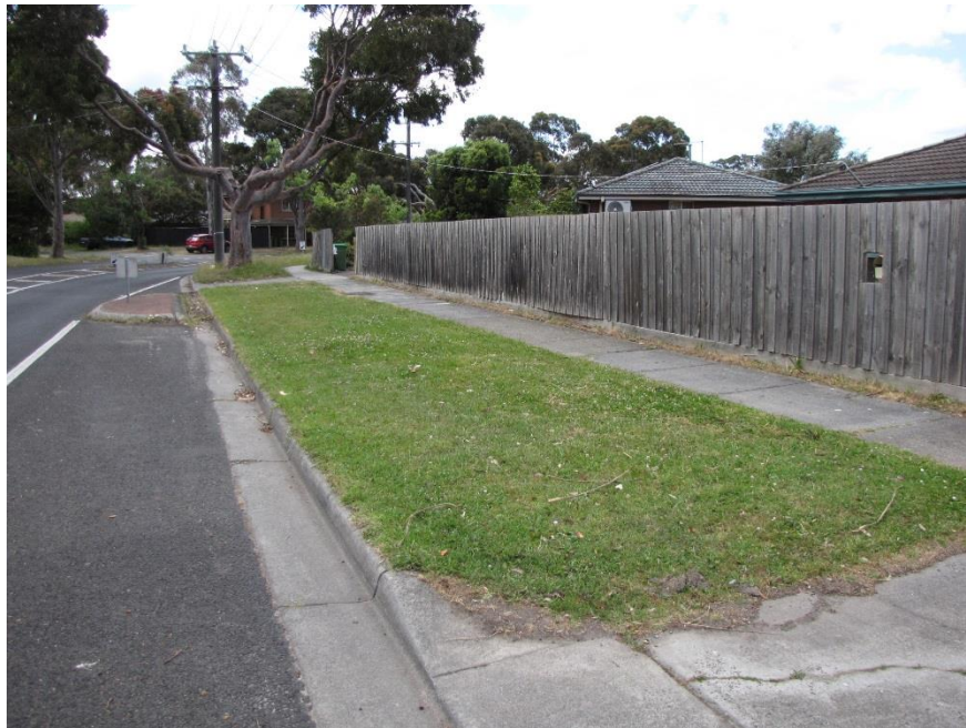
Plate 6 – The Duncan Drive nature strip is clear of existing service pits, utility infrastructure and street trees
