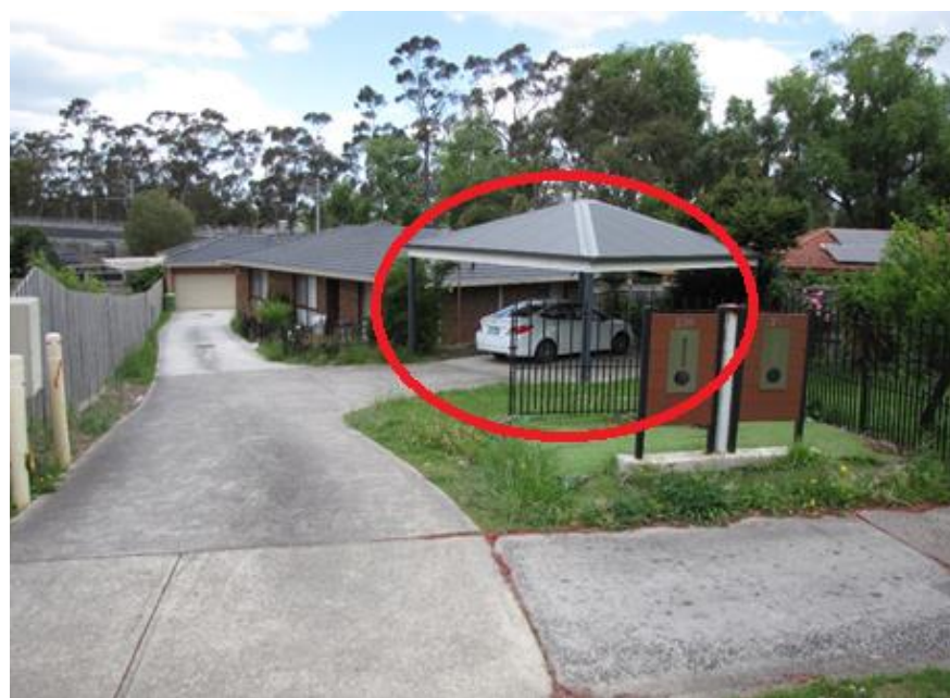
Plate 9 – Example of a double carport in the street setback of a second dwelling development at 130 Duncan Drive
