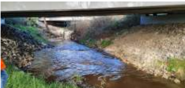
Figure 7. Upstream portion of Toomuc Creek under Princes Fwy bridge
