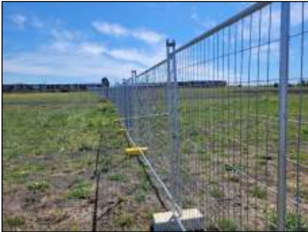
Plate 1. Example of suitable temporary protective fencing.
