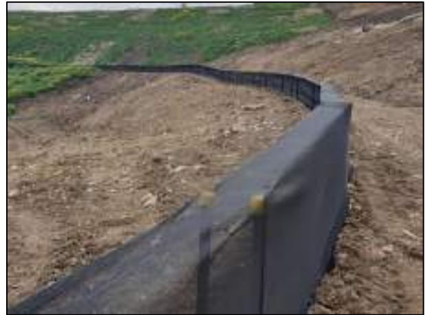
Plate 2. Example of suitable frog silt fencing.
