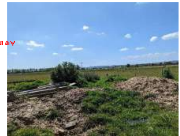
Photo 24: Additional stockpiles of soil and debris at rear of property at 26A Enterprise Rd.
