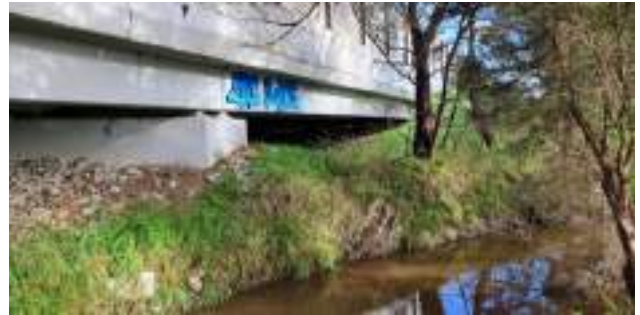
Figure 6. Upstream side of the Princes Fwy bridge
