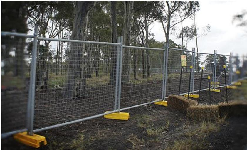
1. **Protection Barrier:** A protection barrier shall be set up around the trees to be retained. The fencing material is to be constructed of a galvanized steel mesh type of material. Fence height 2.1 metres. Concrete filled blow moulded fence feet are to be used as a base support so no protrusion into the soil will take place.
