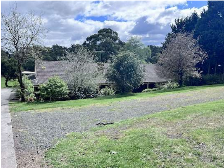
Front of current dwelling, existing concrete & gravel driveways
