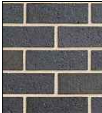
(A) EXTERNAL BRICK WALLS- GREY
