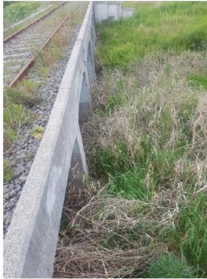
Figure 5: Upstream side of Southern Boundary drain flowing through disused railway culvert
