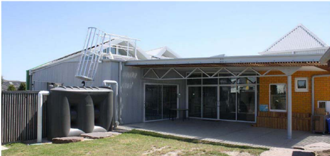
Figure 5. Arena Family and Child Centre rainwater tank
