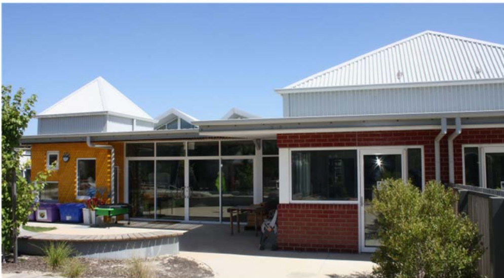
Figure 4. Arena Child and Family Centre northern facade
