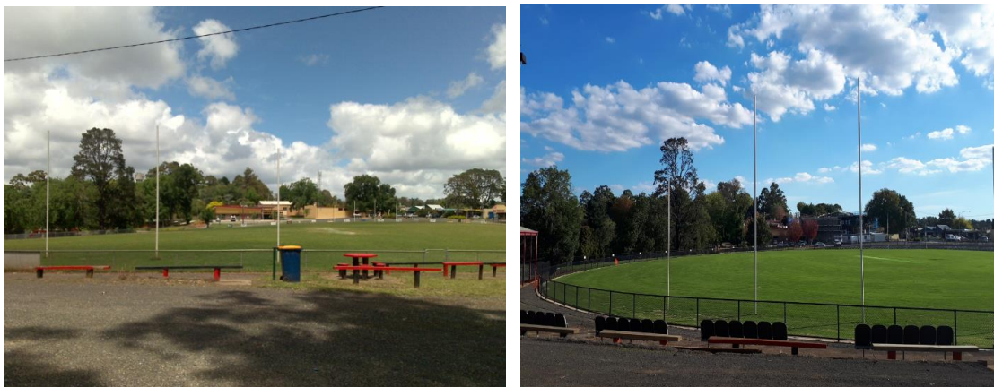
Worrell Recreation Reserve Oval (before & after re-construction)
