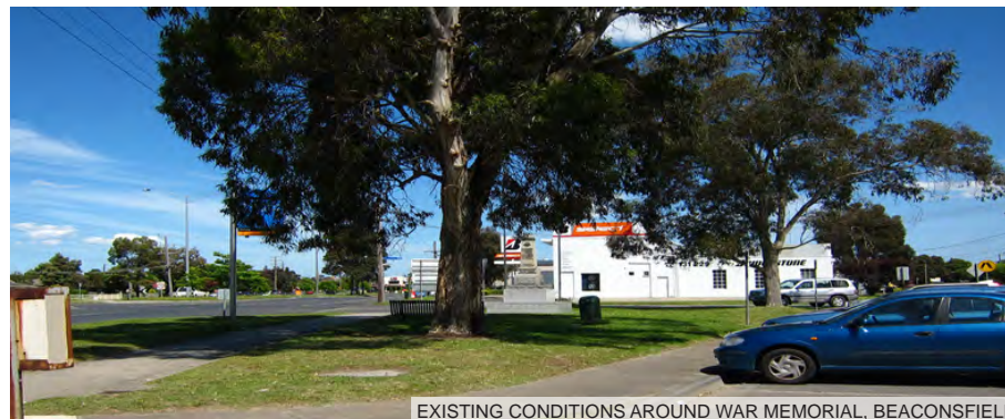
EXISTING CONDITIONS AROUND WAR MEMORIAL, BEACONSFIELD
