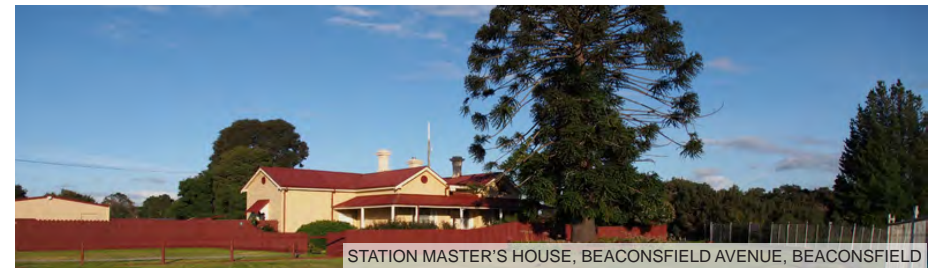
STATION MASTER'S HOUSE, BEACONSFIELD AVENUE, BEACONSFIELD
