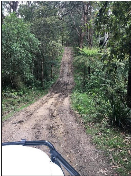
Image 3: Halifax Road, Nar Nar Goon. Note encroaching of verge (horizontal) and overhanging (vertical) vegetation
