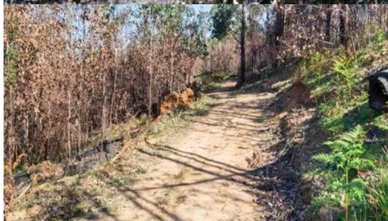
Figure 4. Example of a tanker compliant Fire Access Track.
