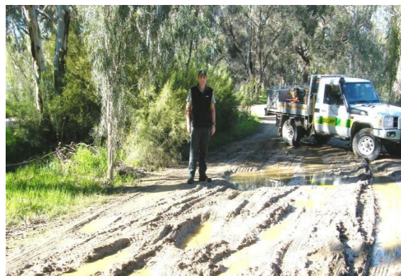
Figure 6. Damage from illegal woodcutters to a Fire Access Track.
