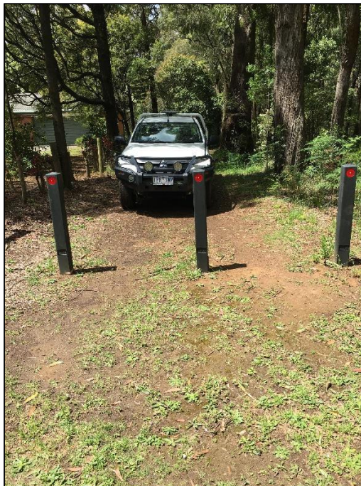
Image 2: Clematis Park Road, Emerald. Note installation of bollards at reserve entrance
