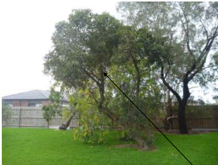
Tree in Question Showing Overall Poor Structure
