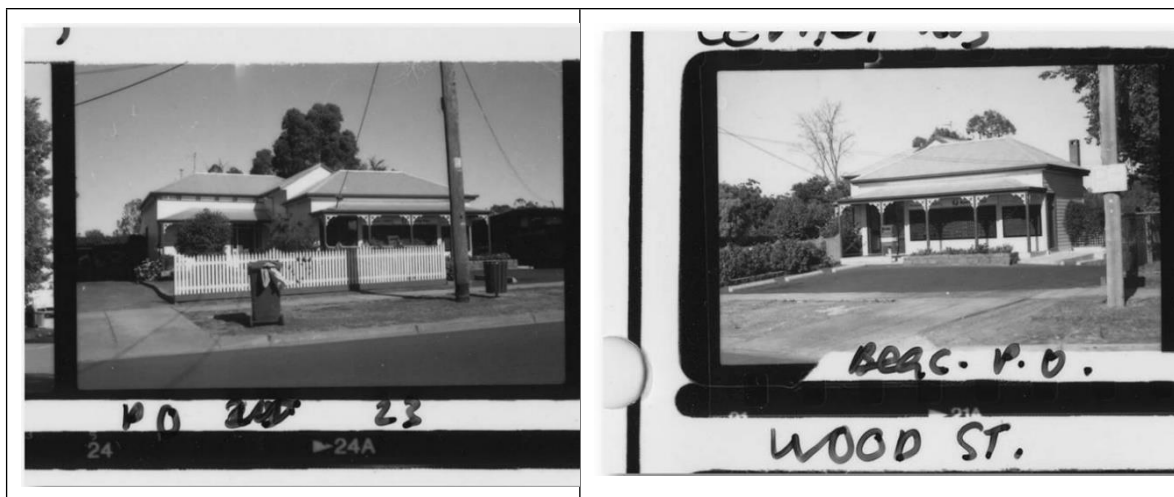
Figure 3: Additions to the front façade as seen today (Photo dated post April 1992)
