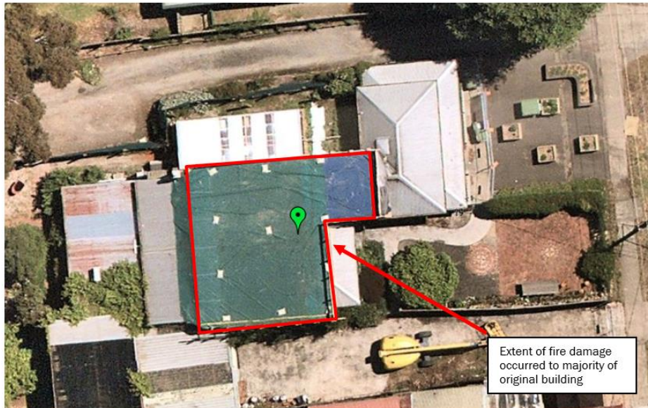
Figure 5: Extent of fire damage to buildings (NearMap image dated 25 Nov 2020)
