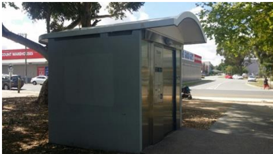
109089 Pakenham Bourke Park Exeloo
