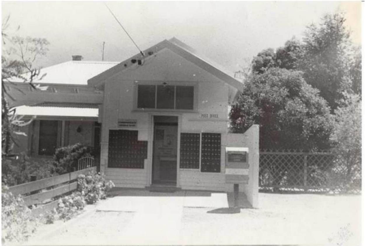
Figure 2: Former Beaconsfield Post Office taken from Beaconsfield Progress Association website (circa 1988)
