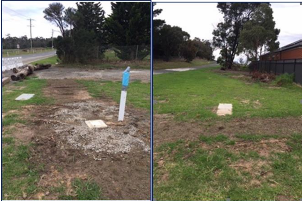
Figure 6. Services in Mulcahy Rd at Thewlis Rd
