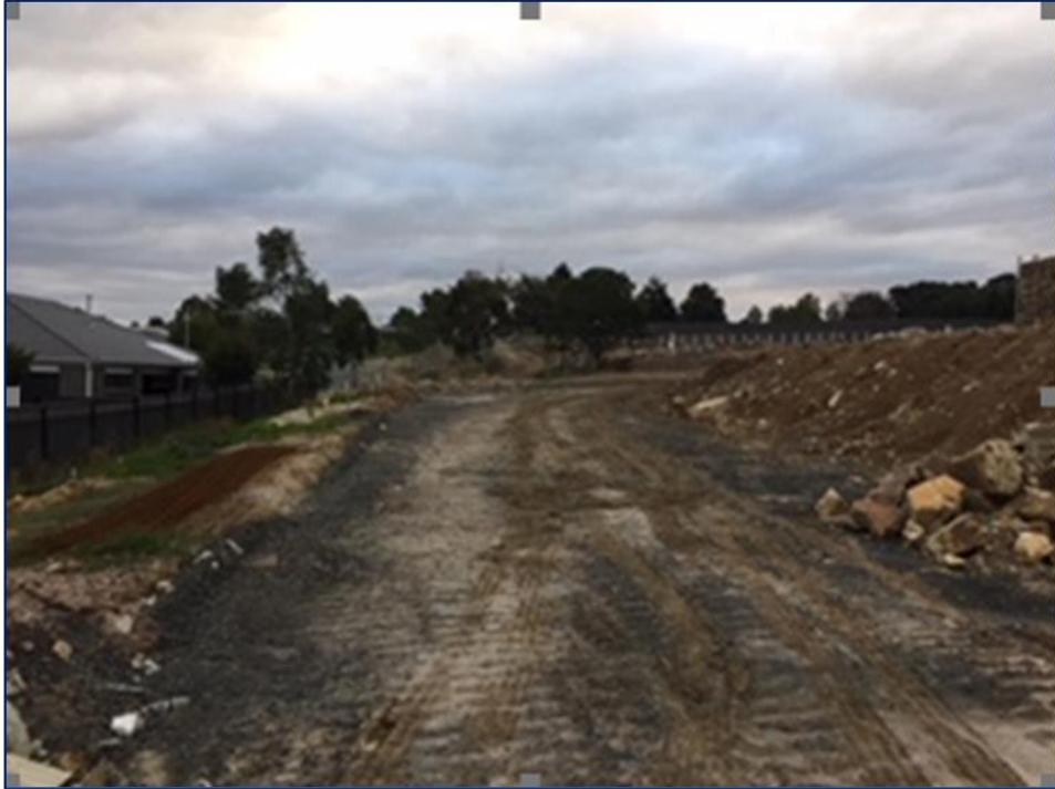
Figure 5. Mulcahy Road looking west to Moritz Street from Pointer Drive- soon to be constructed by developer
