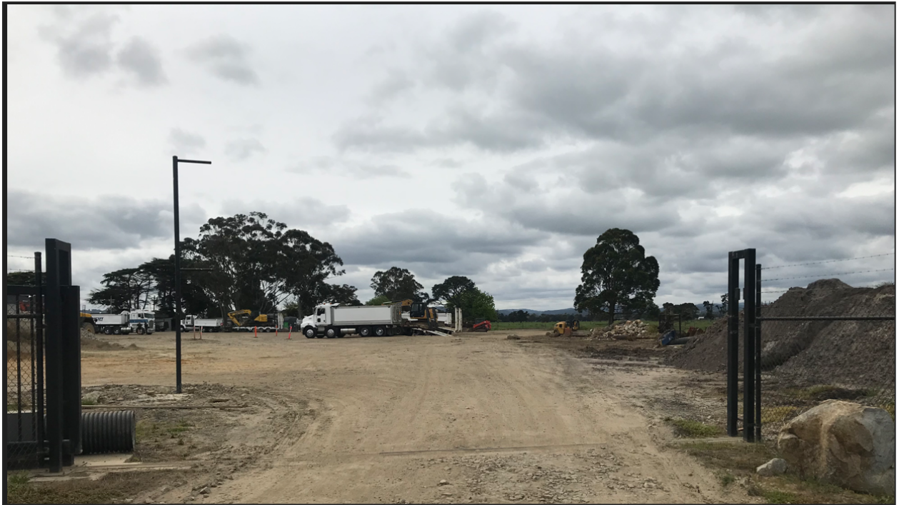
Image 2: Subject site – view from McCraws Road
