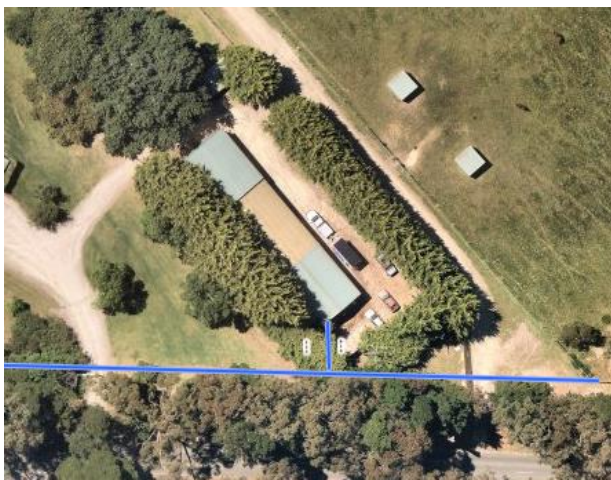
117 Split Rock Rd Upper Beaconsfield 8.0m to the road boundary
