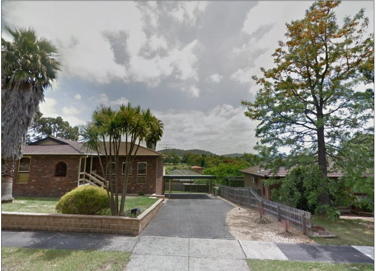
Figure 17 – Typical development of The Ridgeway to the south of the subject site (Google Streetview, Feb 2023).
