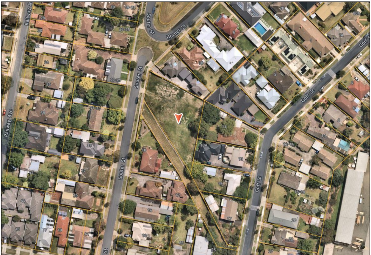
Figure 1: Aerial view of subject site (NearMap Feb, 2023)
