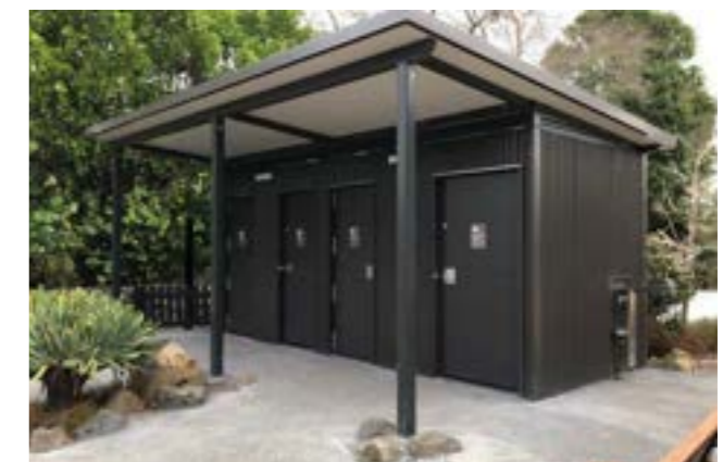
Automatic, DDA compliant toilet unit with unisex, ambulant and disabled cubicles. Consider Colorbond cladding or similar that blends into the environment
