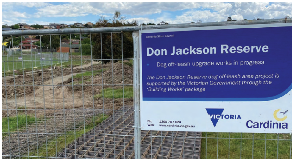
Figure 14: Don Jackson Reserve, Pakenham, Dog off leash area under construction
