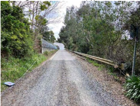
Existing unconstructed Road
