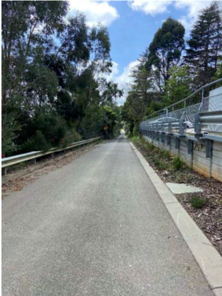
Adjoining constructed Road (typical construction)
