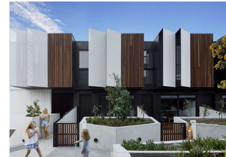
Image 13: Benchmark imagery of 2 storey attached residential townhouses typology (Source: Roseneath Street, Victoria)
