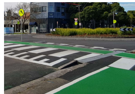
Image 33: Benchmark imagery of raised pedestrian crossing including bike crossing (Source: Moray and Dorcas Street, South Melbourne)
