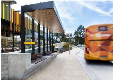
Image 23: Benchmark imagery of bus exchange with adequate seating and weather protection (Source: Rosanna Station, Rosanna)
