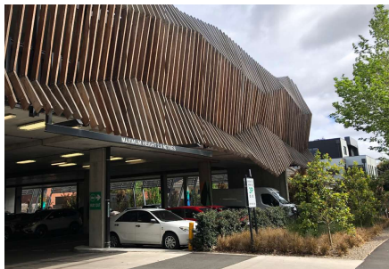
Image 30: Benchmark imagery of sleeved car park with architectural treatments (Source: Atkinson Street Car Park, Oakleigh)
