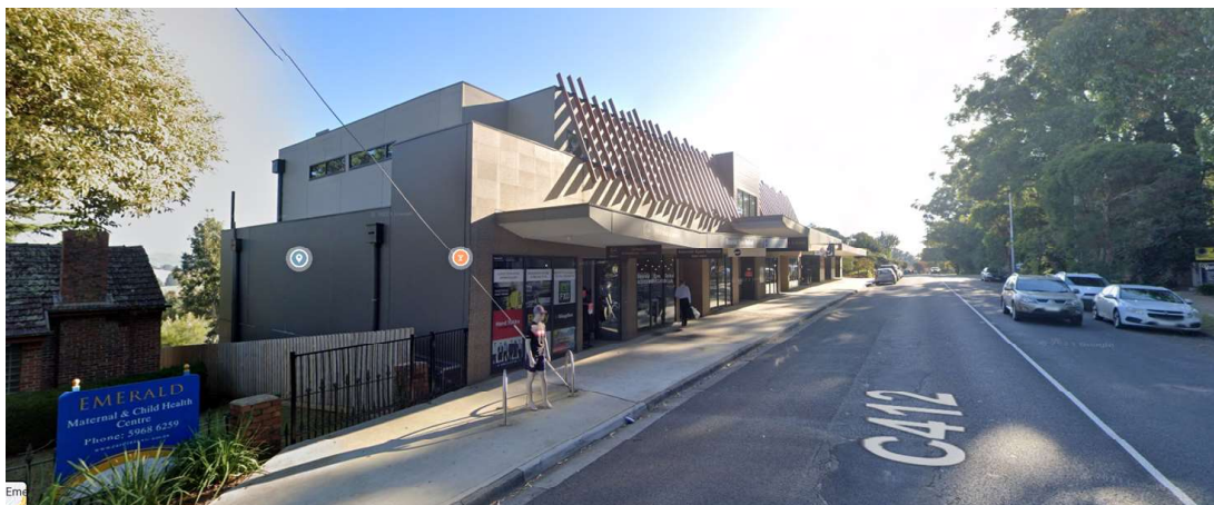
Figure 8 - Existing streetscape and recent double-storey development to the west of the subject site.
