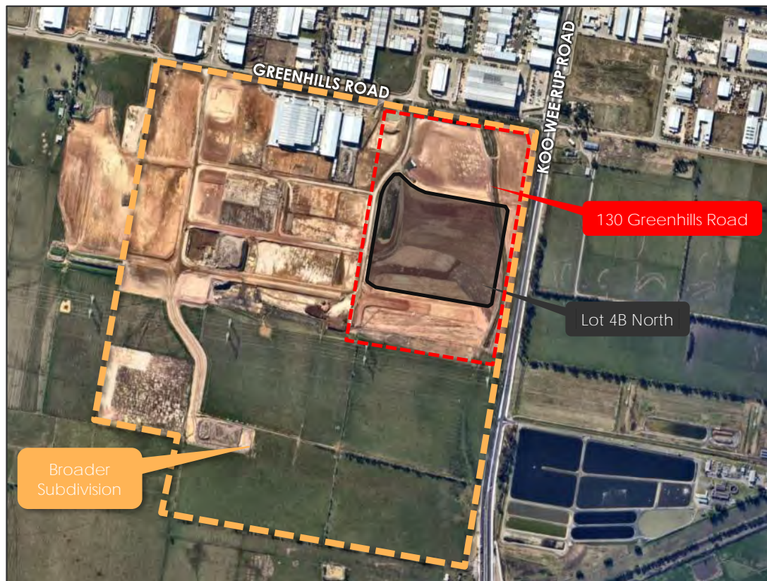
Figure 2 Site Context (1 August 2024)
