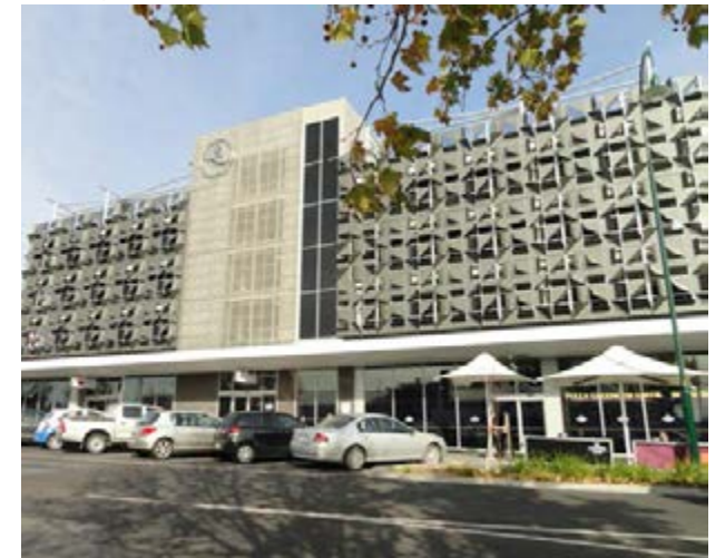
Multi deck car park with mixed use at ground level, Bendigo *
