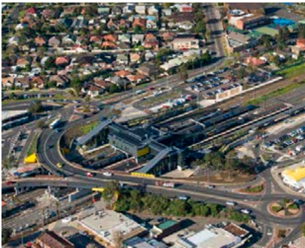
Aerial view showing extent of the Sunshine Railway Station redevelopment, [Photo: Courtesy of the RRLA]
