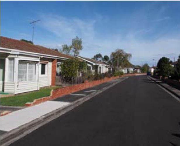
Saint James Aged Care Estate has potential precinct heritage, Dame Pattie Avenue
