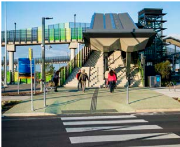
West Footscray railway station was rebuilt 160 m west of old station [Photo: Courtesy of RRLA]
