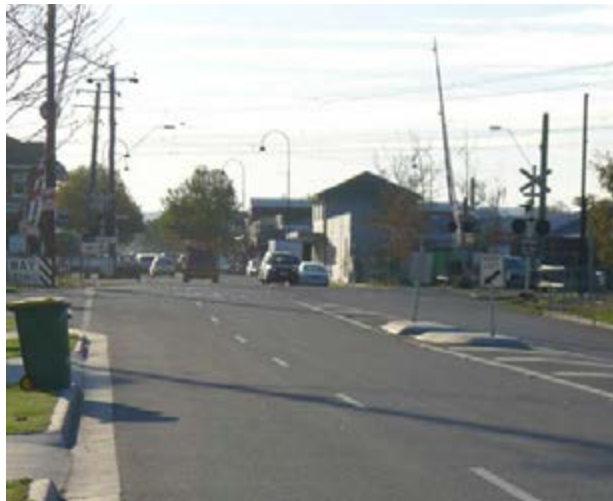
Level crossing at Main Street, Looking from Bald Hill Road
