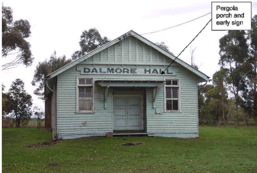
Figure 1 view from road
